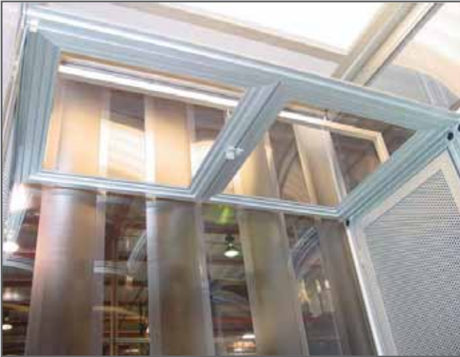
EasyStreet used AirBlock™ isolation components from Simplex® to create a shell enclosure around the colocation cabinets.
